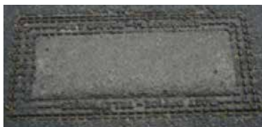
Old style cast iron and concrete 38x80cm
